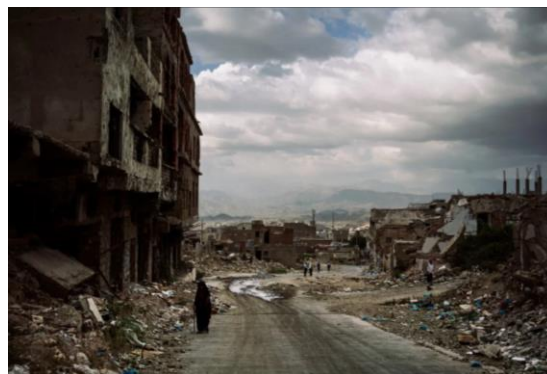
Fig. 14 Structures in the al-Jahmaliya region of Taiz have been decreased to rubble
